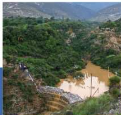
Fig. 2. Traditional rock dams filter water and simultaneously allow infiltration. © Raúl Hernández Garcíadiego.
