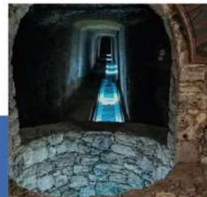
Fig. 4. Water spring linked to a system of well and seeping galleries ( galerías filtrantes ). © Raúl Hernández Garcíadiego.
