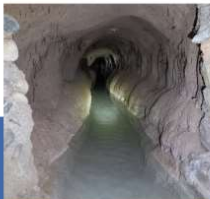
Fig. 1. Hand-dug 'galería filtrante' (seeping tunnel) collects water for irrigation. © Raúl Hernández Garcíadiego.
